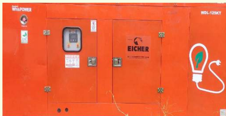
Diesel Generator Set (125 kVA)
